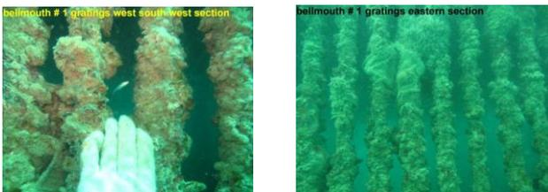
Figure 2. Fouling on the bar rack at a sea water suction bellmouth
